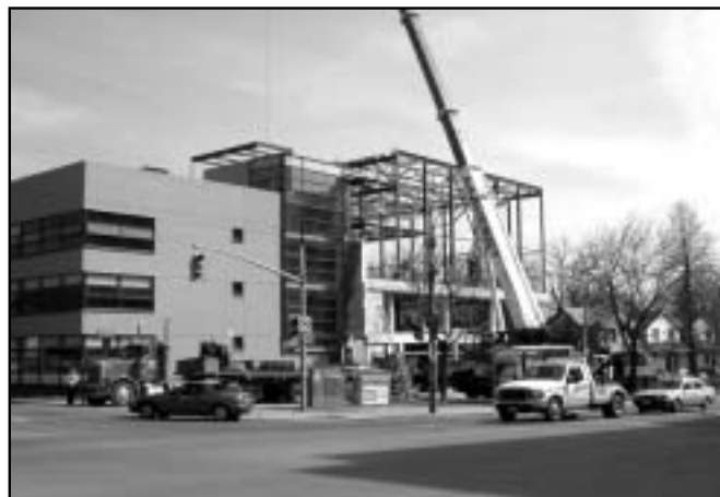
“HEY MAC, WHERE YOU WANT ME TO PUT THE TETHERBALL?” Greenwood College School has remained true to its Kilcoo “authenticity” ethos, as Phase II construction continues on schedule.
